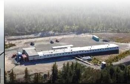
Initial Construction Starter Camp *installed septic
