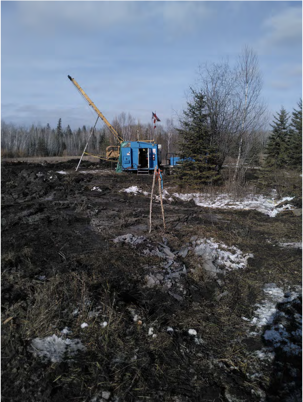
Figure 41. Set for A20-11 and 12 with A20-13 underway
